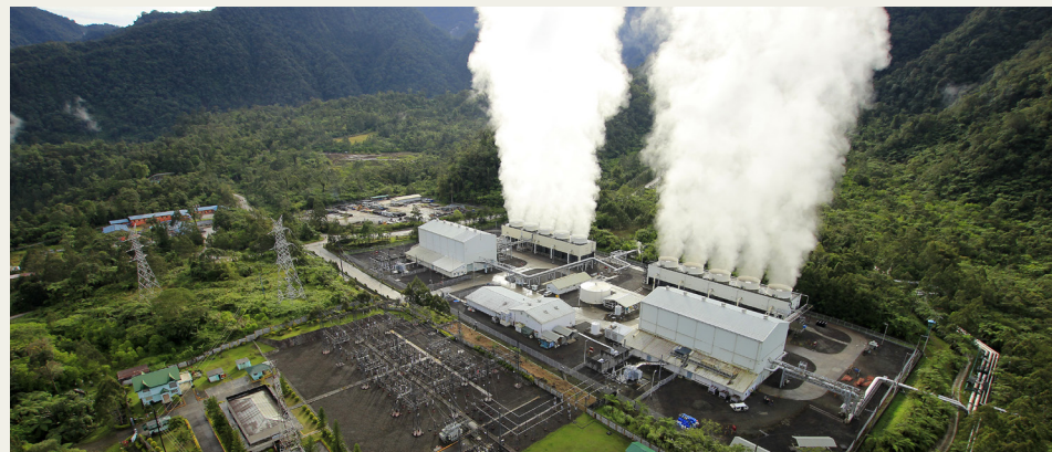
Energy Development Corporation's Geothermal Plant in Mindanao, Philippines
