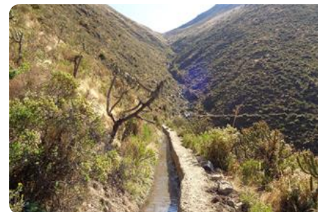
8.4 km long infiltration channel in the Andes Mountains 12
