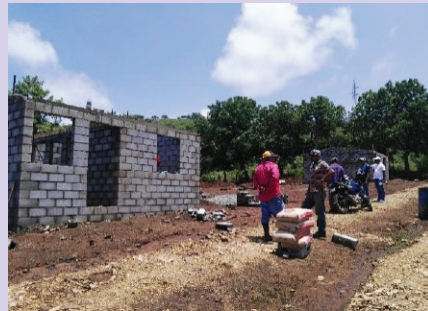
Building a new house in Nueva Jerusalén.
