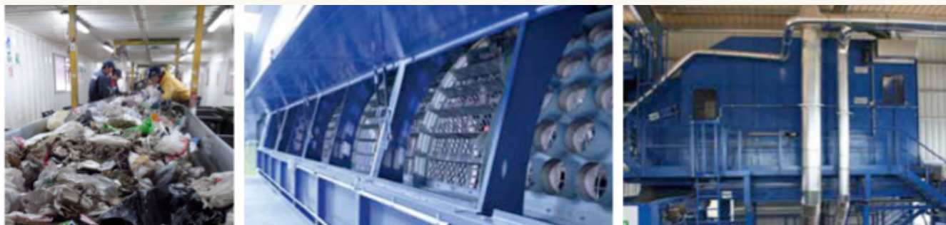
Figure 19: Manual Sorting Table, Trammel, and Air Separator
